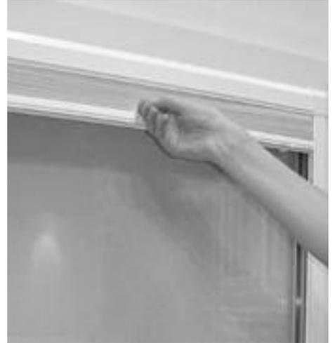
2. Release the frame from each bracket by inserting a flat headed screw driver into the hole and depress against the lip of the brackets.
